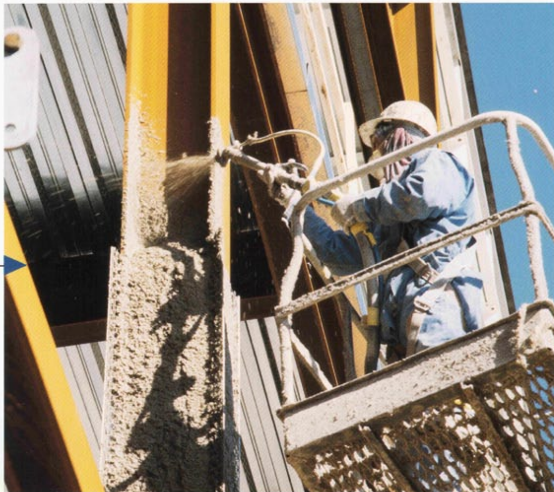
Monokote Type Z-146 application in progress at Malden Mills.
