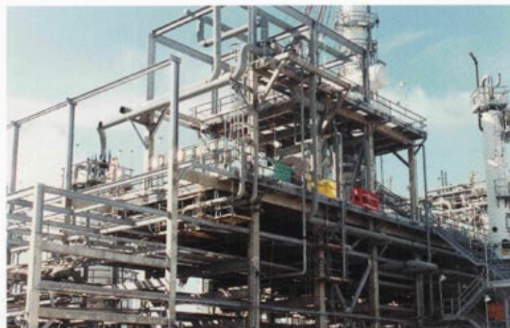
Monokote Type PK-150 provides tough, rugged fire protection for OxyMar's new vinyl chloride monomer plant in Ingleside, Texas.
