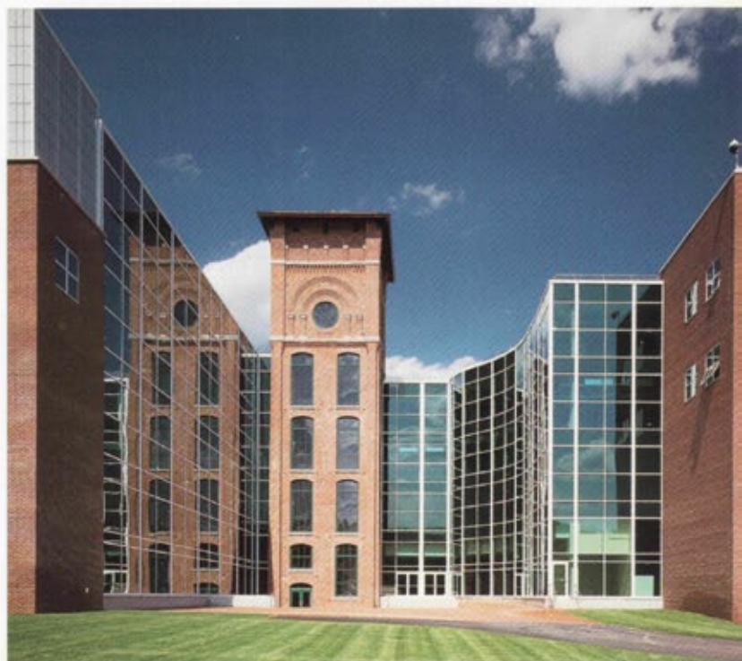
Newly reconstructed Malden Mills manufacturing facility.
