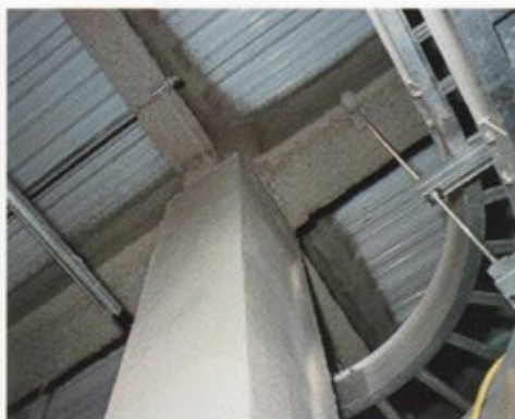
Monokote Type Z-146 boxed and trowelled at Rhode Island's Narragansett Electric co-generation plant.
