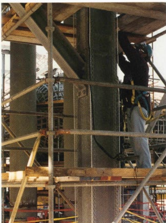
Monokote Type PK-150 provides tough, rugged fire protection for OxyMar's new vinyl chloride monomer plant in Ingleside, Texas.
