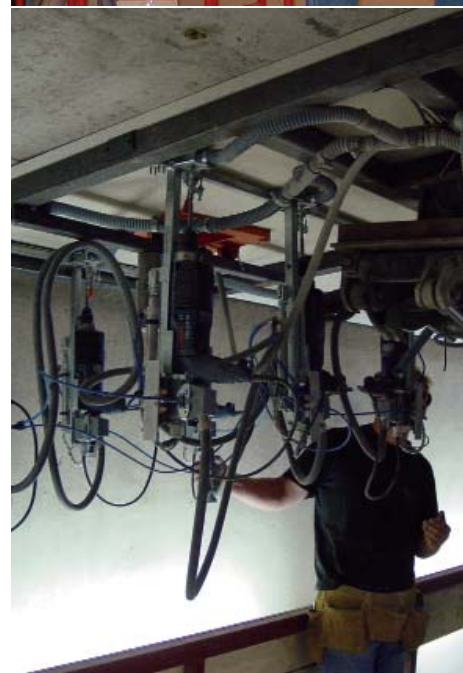
FIGURE 47 (above and this pictures) : DRILLING OF CONCRETE
